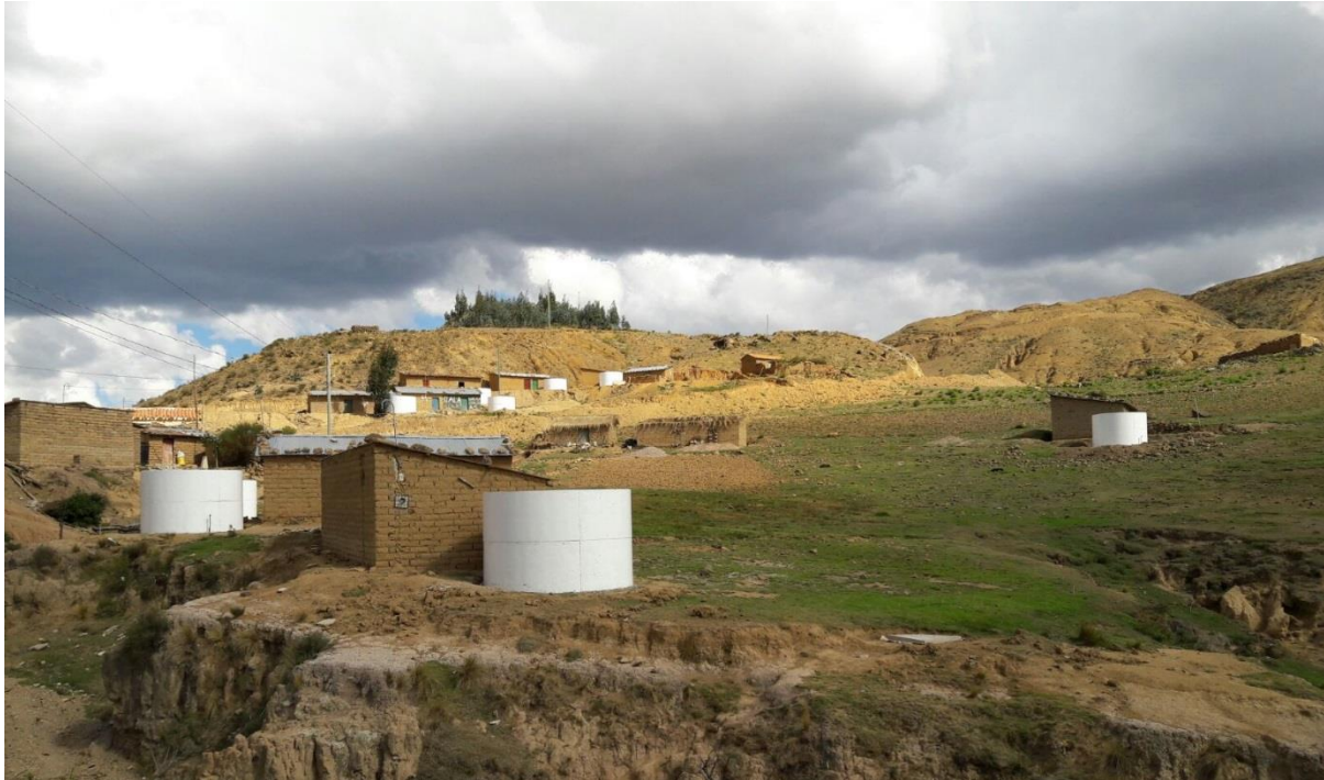
Figure 7 – Rainwater harvesting tanks built by Don Goyo Ecotechnology Company in the Department of Potosí, Bolivia (Courtesy of Don Goyo Ecotechnology Company)
